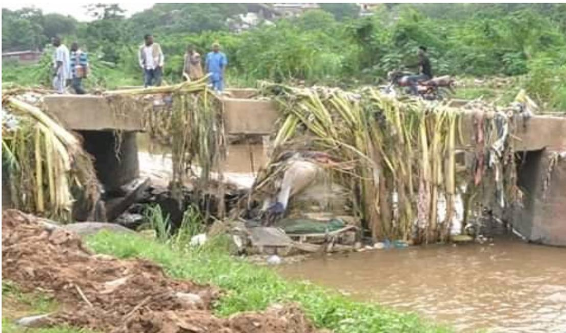
**Figure 5: Blockage of River Channel with solid wastes**
